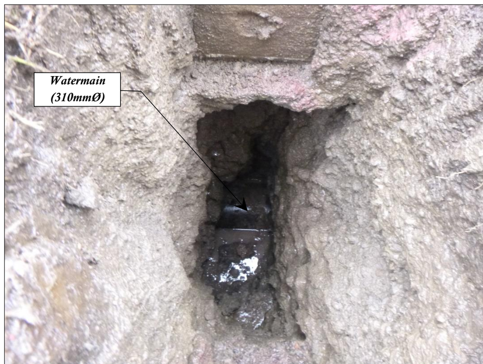
Figure 4 – Exposed structure
