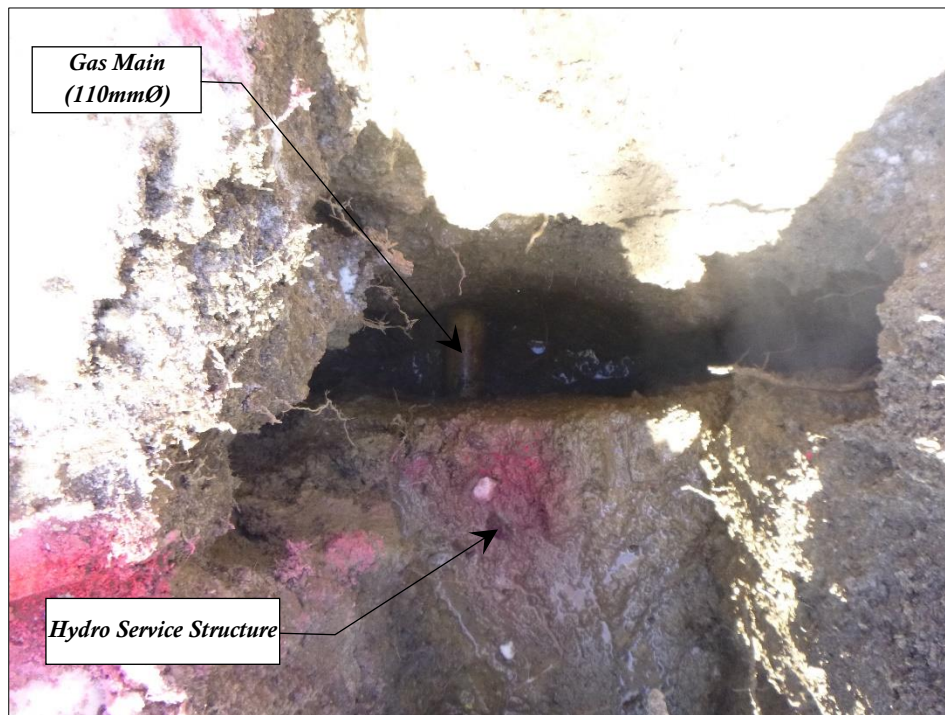
Figure 22 – Exposed structure
