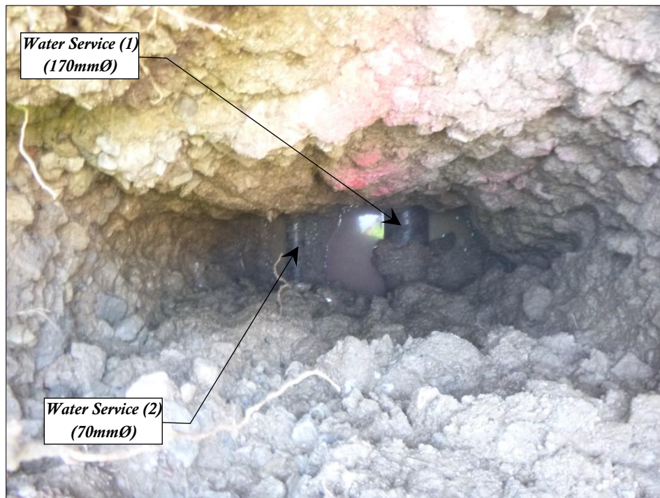
Figure 34 – Exposed structure
